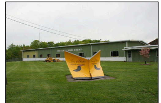
Above (top to bottom): Town Hall on Kings Highway, which houses the Town supervisor and Town Board offices, Town clerk, assessor and police department; Town Hall sign; and Town highway department on Laroe Road.
