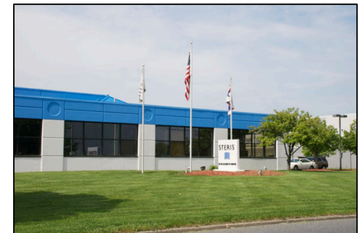
Above (top to bottom): The Shortline Bus garage during construction in the summer of 2013; Iron Mountain within the Village of Chester’s industrial park; and Steris Corp., which is also situated within the Village of Chester industrial park on Elizabeth Drive. This Plan supports the creation of a diverse economic base, including light industry.
