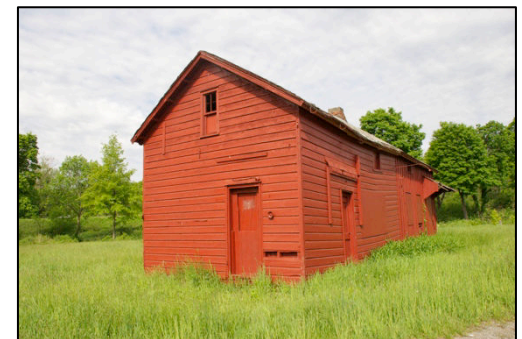
Above (top to bottom): Barn at Fury Brook Farm, which was converted to light industrial use; Laroe Saw Mill at the corner of CR 13A and CR82 Bellvale Road; and small barn across from Brookview Farm on Route 17M. There is a growing niche agricultural sector in Chester, which should be supported to save prime farmlands.
