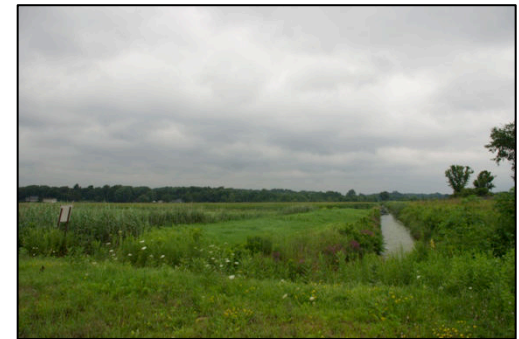
Above (top to bottom): Temporary pumping system for canal, which was utilized when pump stations were down (main pumps were down for two years between 2011 and 2013); view of outflow canal as it crosses under Lehigh & Hudson Rail Line and enters Camp LaGuardia; view of canal along Black Dirt field north of the Lehigh & Hudson Rail Line.
